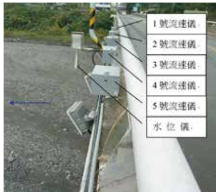
Pingtung Sandimen Bridge
